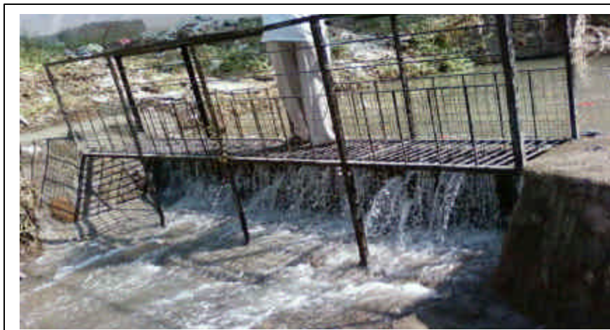
Cleaning of solid waste and debris from the Nalla course
