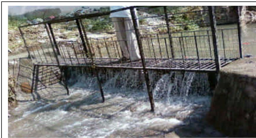
A metal Screen was fitted to trap the solid waste and then Green Bridge was installed. After one Green Bridge, there was considerable reduction in the COD level. When sample was taken after second Green Bridge for analysis, the COD was reduced to 81 mg/l from initial 270mg/l. Local trees, bushes are planted along the banks of the nalla and many species are naturally growing there increasing biodiversity.
