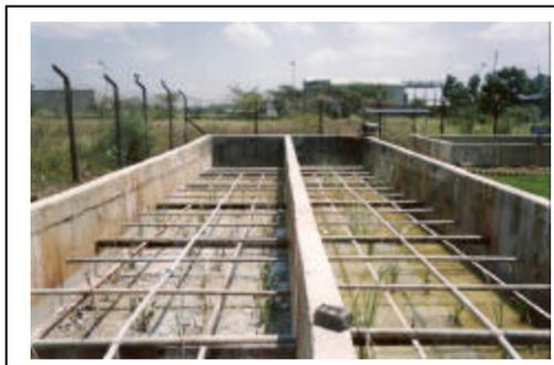
View of the Soil Scape Filter without plants. Wastewater is distributed on the top of Ecofert layer using grid of pipelines.
